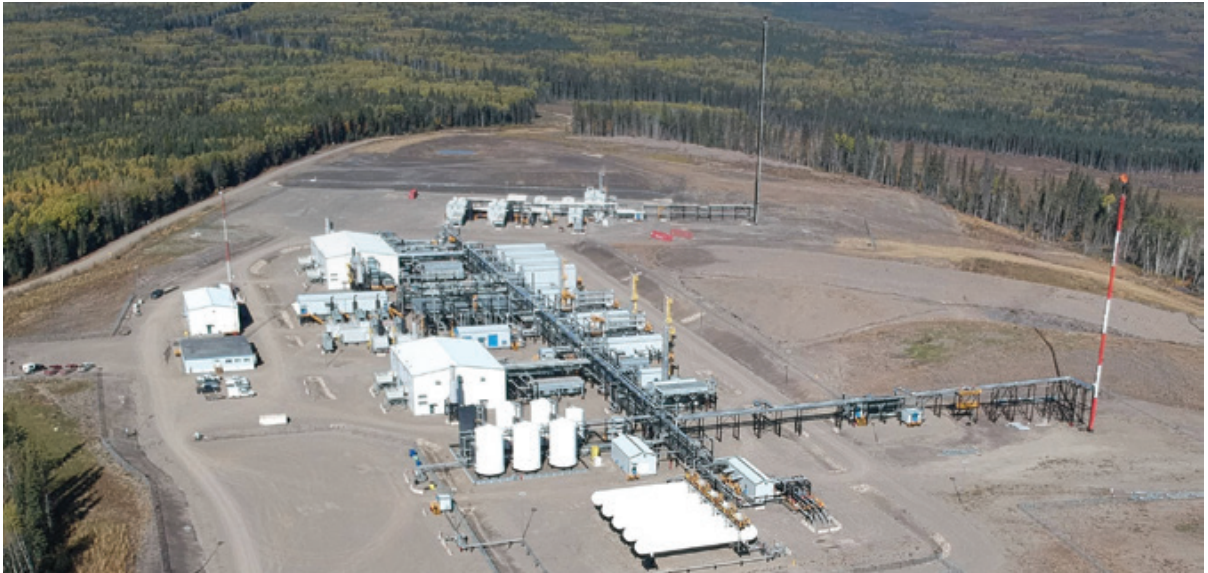
In August 2018, we announced an agreement with Kelt Exploration Ltd. to provide energy infrastructure for the liquids-rich Inga Montney development. This underpins the expansion of the Townsend complex, including the addition of a 198 MMcf per day C3+ deep cut gas processing facility.
