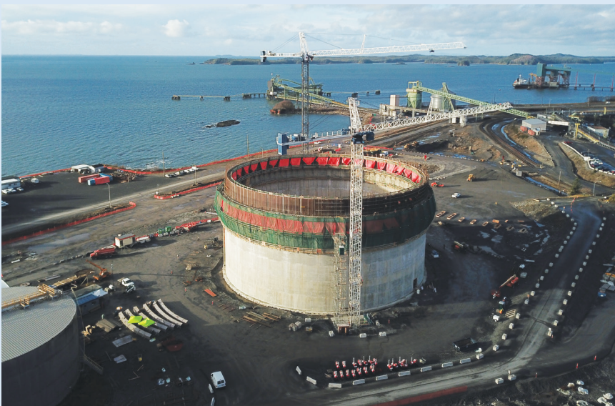
December 6, six of eight concrete pours are complete on the outer wall of the propane tank
