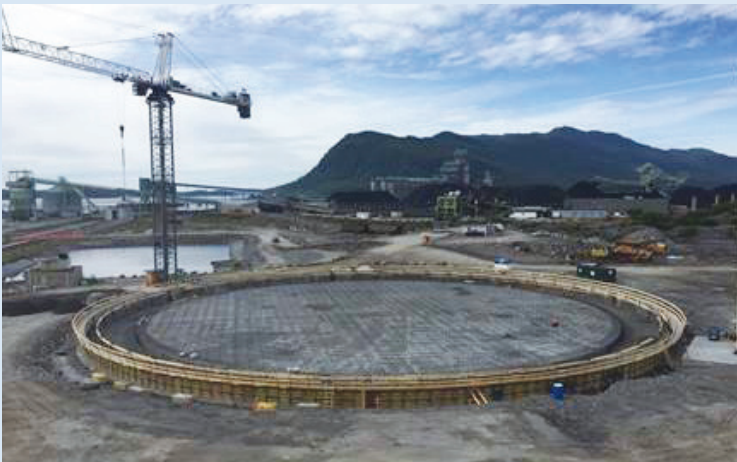
June 26 – installation of rebar on the propane tank
