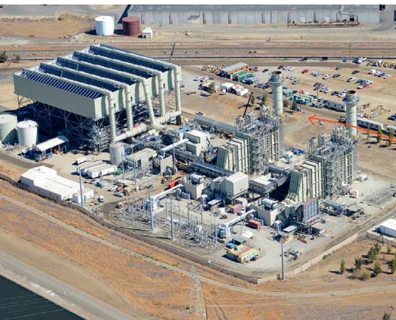
The Tracy Combined Cycle Power Plant is a 330-megawatt, natural gas-fired power generation facility located approximately 97 kilometres east of San Francisco in the San Joaquin Valley owned 100 per cent by AltaGas.
