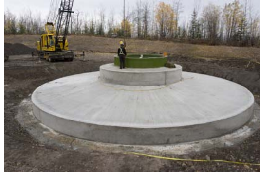
Completed turbine foundation
