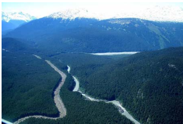
Access road with transmission line route and with Iskut River
