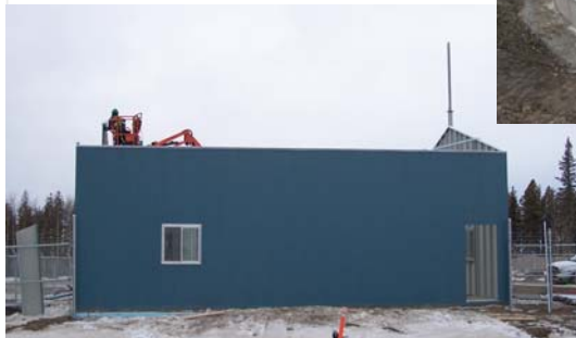
Substation under construction, February 2009
