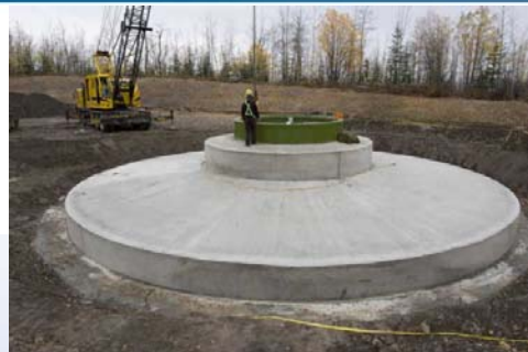
Completed turbine foundation, October 2008
