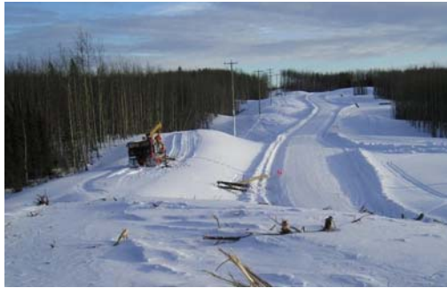
Transmission lines, January 2009
