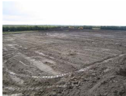
Acme plant site cleared for construction
