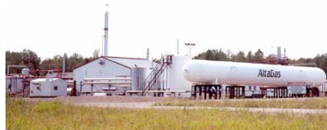
Sylvan Lake gas plant
