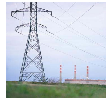
Sundance B power plant
