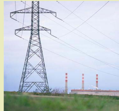
Sundance B power plant
