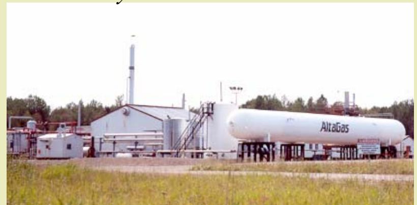
Sylvan Lake Gas Plant
