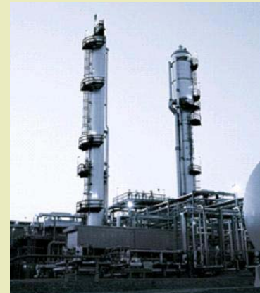
Joffre Ethane Extraction Plant
