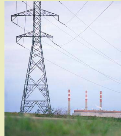
Sundance B Power Plant
