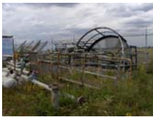
Caged ladder & platform
