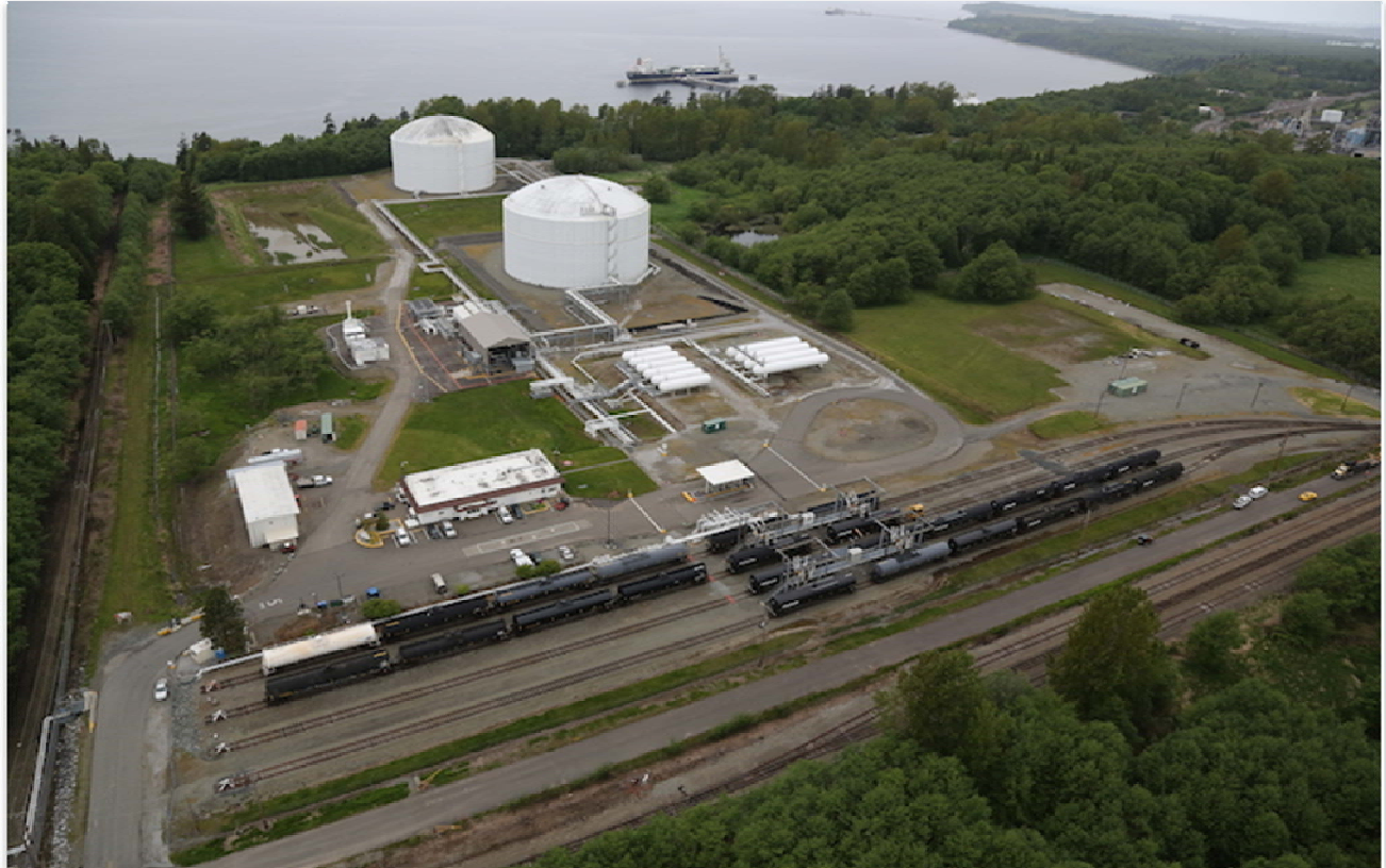
Figure 1-5: Aerial view looking west of Ferndale Propane Export Facility, Washington
